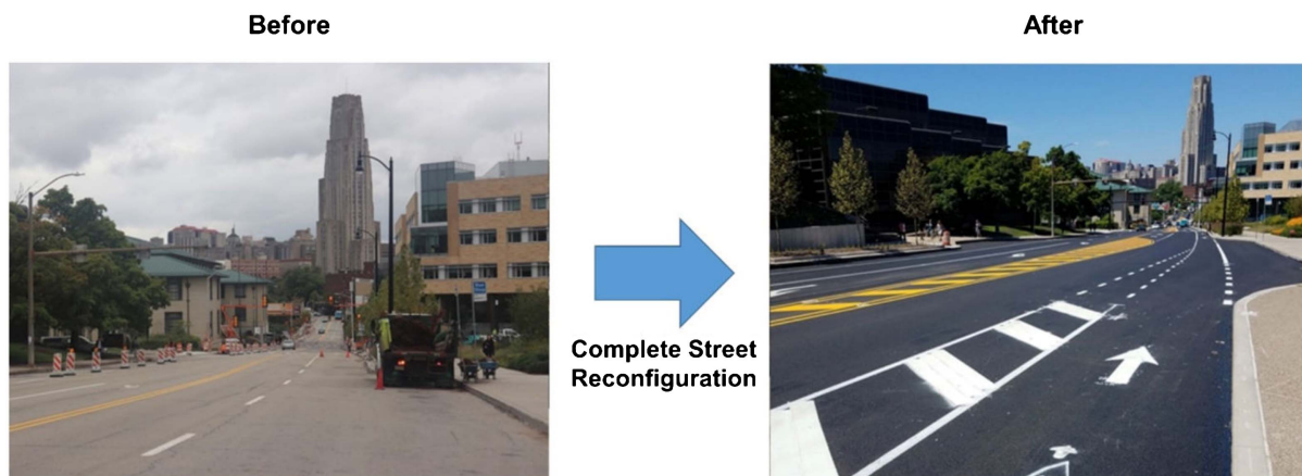
Fig. 2. Forbes Avenue Street configuration pre- and post-retrofit. (Images by Chris T. Hendrickson.)
